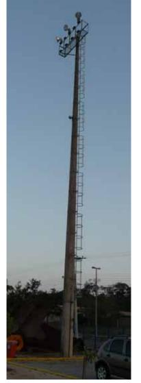
As stated previously each platform could be accessed by a ladder and backscratcher system which would eliminate manriding in the uncertified basket.
