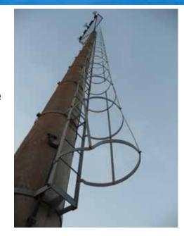
Similarly there was no secondary retention on the light fittings or CCTV cameras installed.
